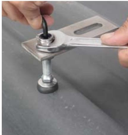
11. Adjusting adapter and tightening it
