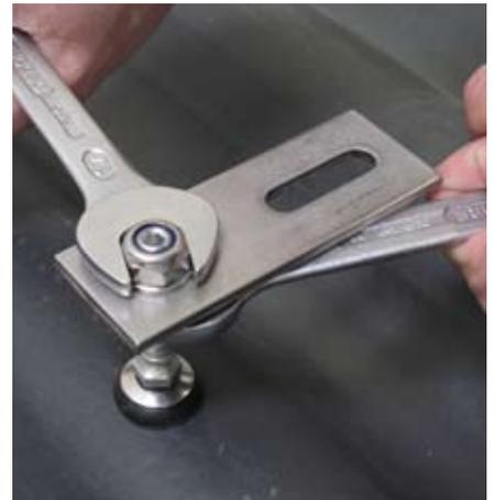
12. The EJOT Solar Fastening is ready installed
