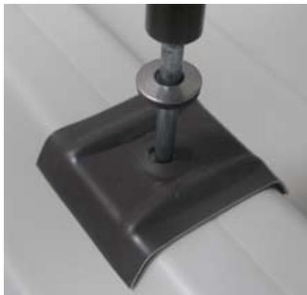
2. Removing sealing washer
