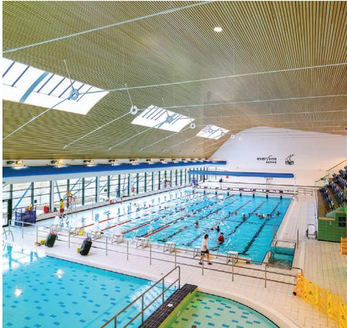
Protektor C5 Coated Profiles are designed to meet the requirements for the suspension and support of boards in High Humidity areas such as swimming pools and wet rooms.
