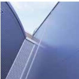
**Sandwich panels** are lightweight steel-faced panels with a core material of stone wool. Paroc panels are used for façades, partitions and ceilings in public, commercial and industrial buildings.
