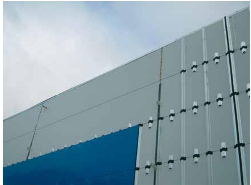
Maximum distance between hat profiles is 600 mm when installed lengthways the panels, and 1200 mm when installed across the panels. In the edge zones the distance is always 600 mm.
