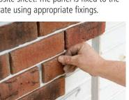
**3.** Brick slips are pushed into place leaving 8-12mm perpendicular gaps between bricks.
