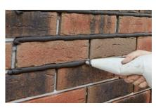
**4.** Specially formulated mortar is then piped into the brick joints.
