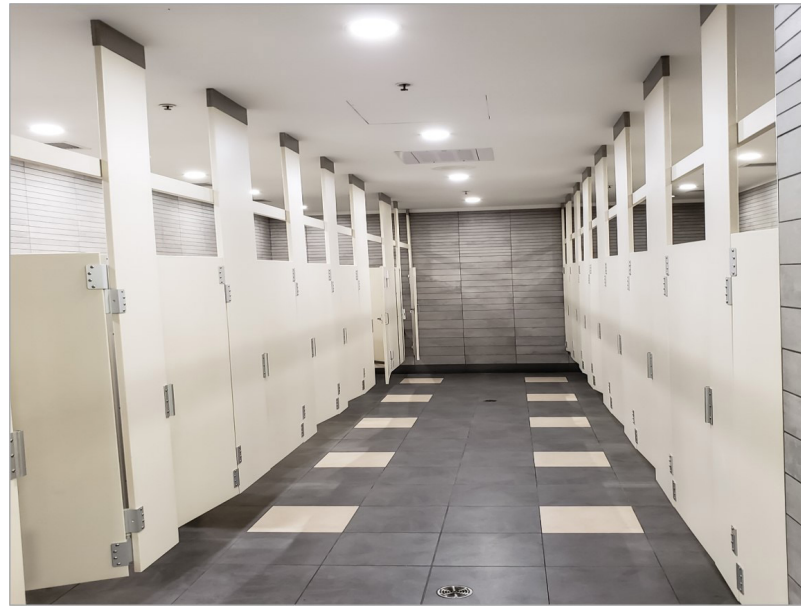
Hadrian Solid Plastic (HDPE), 1400mm Ceiling Hung - w. Stabilizing Bars
