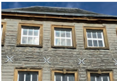
Previously uninsulated frames can benefit thermal upgrading without visual impact
