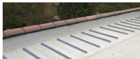
EJObars positioned correctly over membrane strip.
