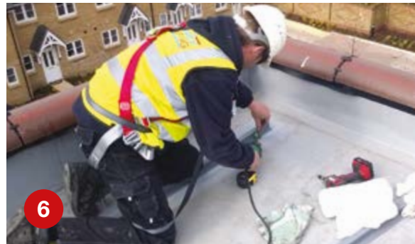
6 Hot-weld EJOBAR in the centre of the reinforced membrane, directly over the line of fasteners.
