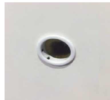
Metal Door Cap removed, Collar exposed
