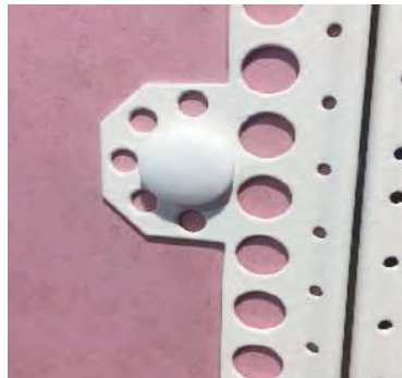
Plaster Board Bung installed
