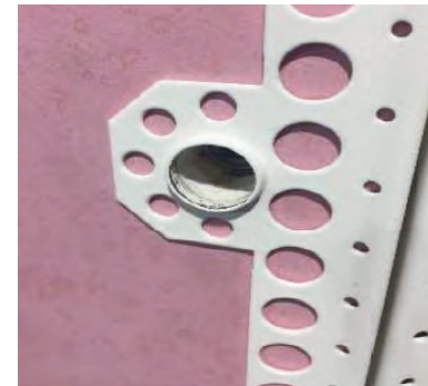
Plaster Board Bung Removed
