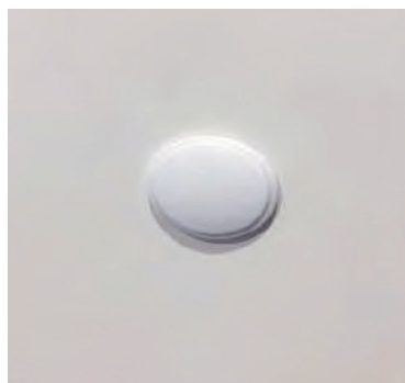
Metal Door Cap & Collar installed
