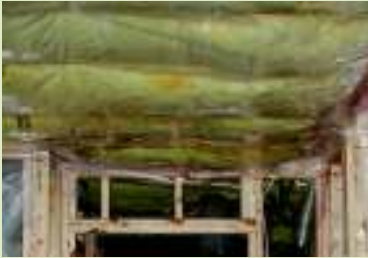
A continuous air barrier applied over wood-framing and insulation significantly improves the thermal performance of a building by reducing air leakage.
