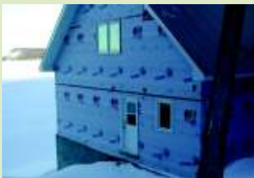
A weather barrier applied to the exterior sheathing prior to siding materials, acts as an additional barrier against wind, rain and snow.
