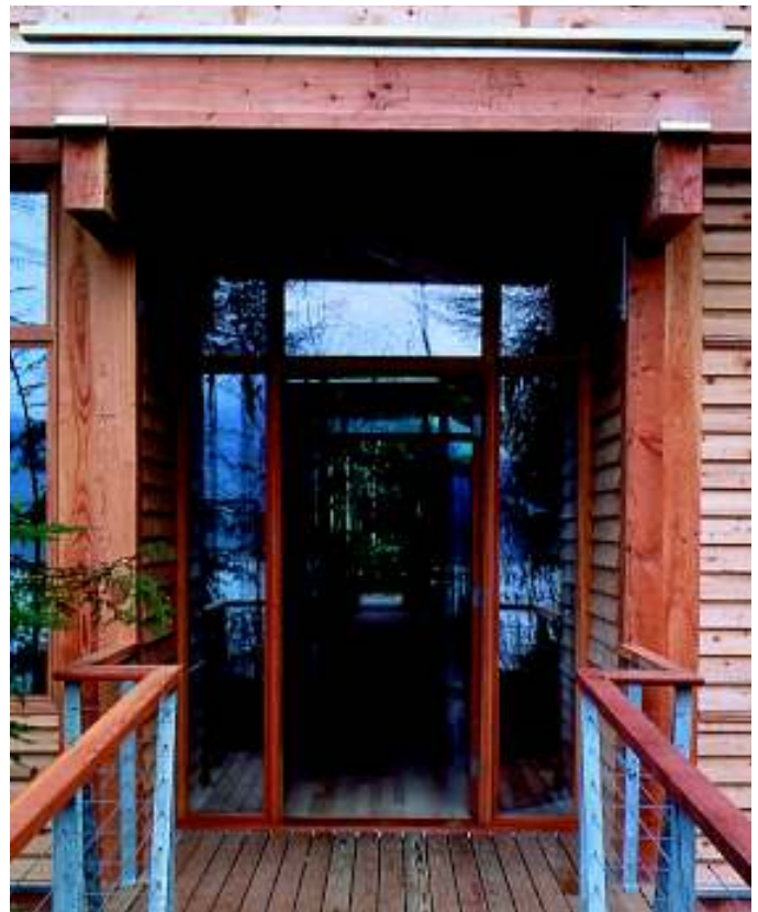
PHOTO 8: Overhangs protect end-grain of beams from moisture.
