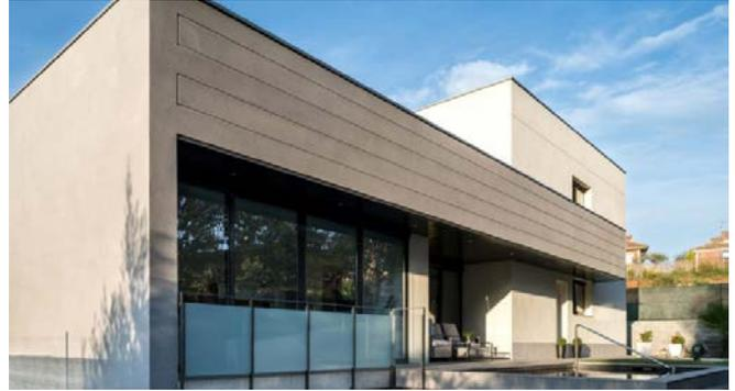
Intercrete 4893 has an equivalent air layer resistance to CO<sub>2</sub> diffusion of 81m
