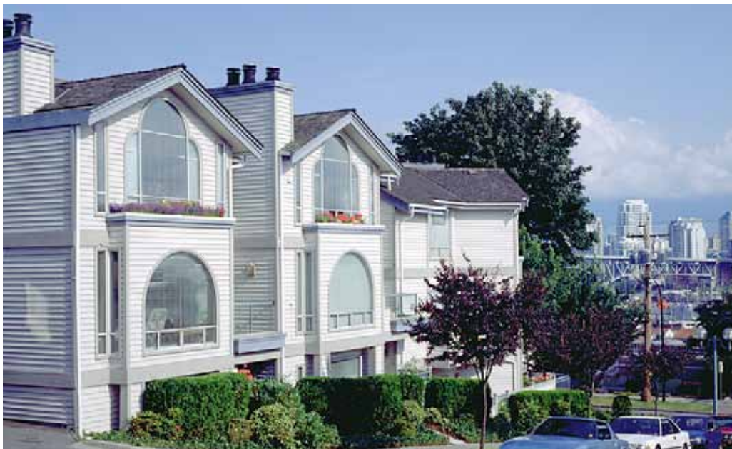
PHOTO 7: The Windgate townhouses near Choklit park in Vancouver, BC use decorative exterior fascia boards at the floor level, combined with sloping roofs and overhangs as part of a moisture management strategy.
