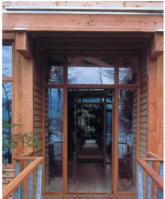
PHOTO 8: Overhangs protect end-grain of beams from moisture.
