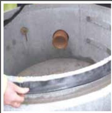
Stretch the seal onto the spigot of the manhole and position it against the shoulder. Make sure the load distributor (the circular part) is located on the upper surface of the spigot.
