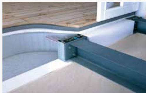
Steel-to-reinforced concrete connection:
