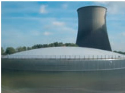
▲ Essent, Maasbracht, Netherlands
