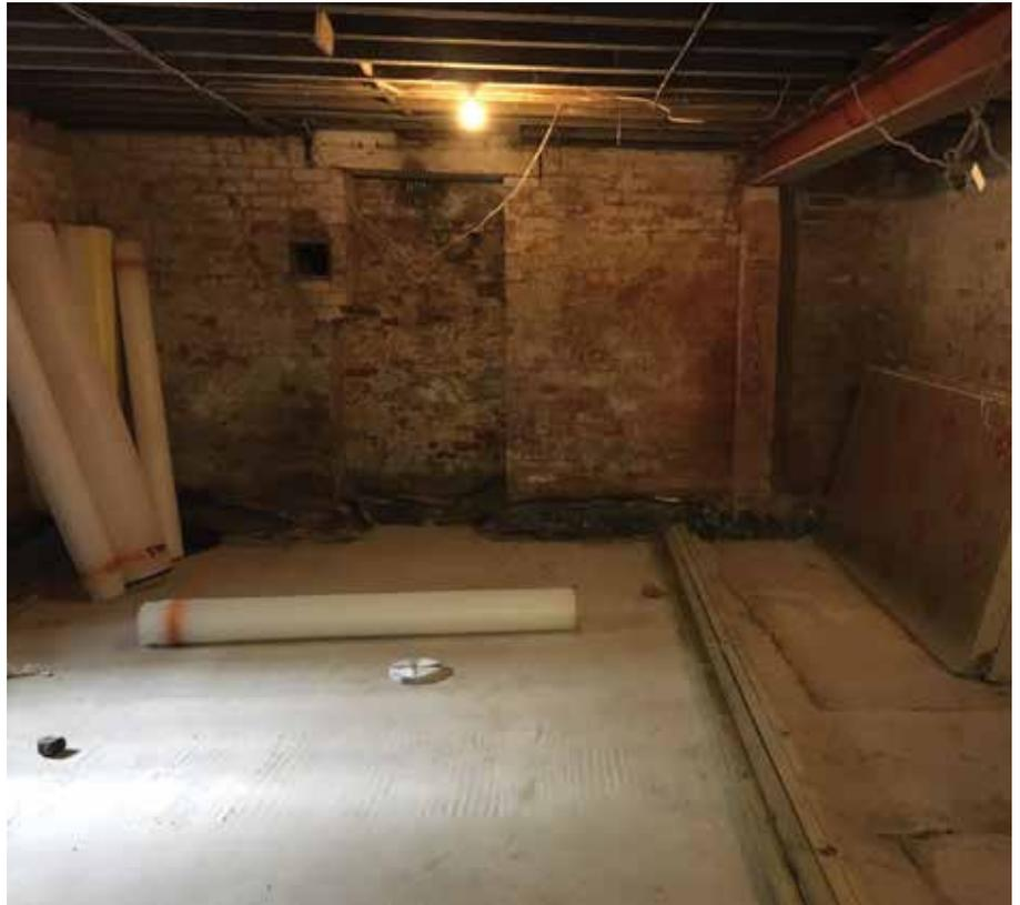
All basements should be constructed (or retrofitted) to cope with groundwater levels up to the full retained height of the basement. Structural waterproofing preserves the integrity of a structure whilst ensuring the usefulness of the building for present and future use.
