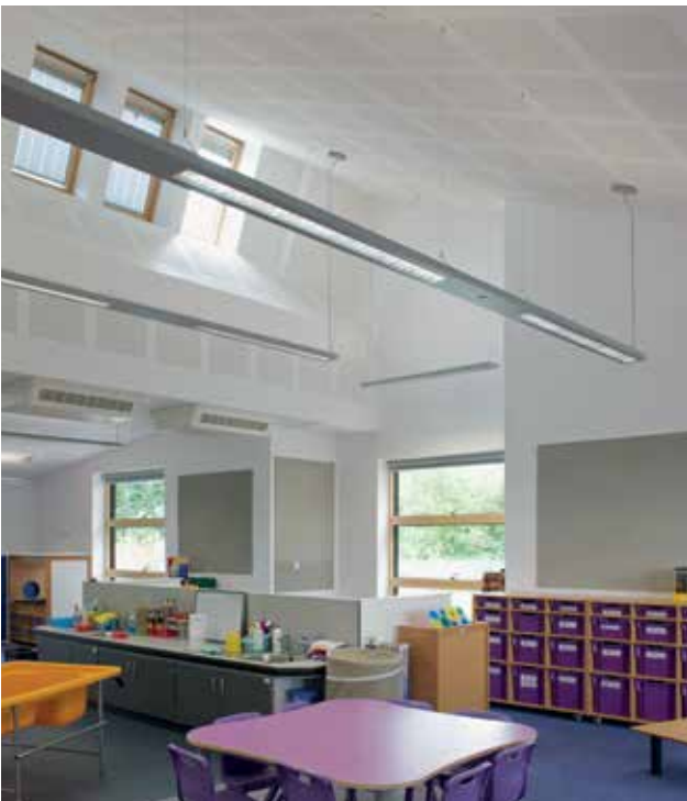
Gyptone QUATTRO 41 board on CasoLine MF frame
