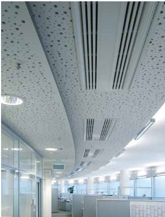
Rigitone 8-15-20 board on CasoLine MF frame
