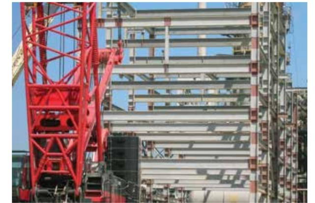
Both flexible and tough, PPG PITT-CHAR XP resists cracking and damage during slinging and handling, so that the fireproof coating remains in good condition when steel is transported and erected on site.
