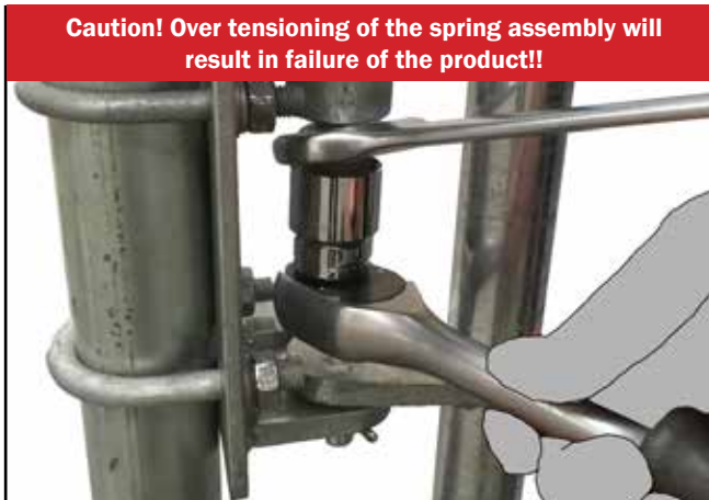
M. Using a 24mm socket & spanner tighten the bolt until the gate completely closes. (You may have to hold the socket whilst using the ratchet). Once the gate is completely closed tighten the locking nut to hold the tension. Caution:- Hold ratchet firmly and do not release until the lock nut is tightened. Repeat as necessary to ensure that the gate closes sufficiently.
