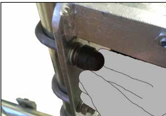
N. Ensure all nuts and grub screws (excluding adjustment screw) on the gate are torqued to 39Nm. Finally, place black caps over nuts. Ensure that the structure to which the gate is attached to is sturdy, does not rotate and nuts and grub screws are torqued as per manufacturers guidelines.
