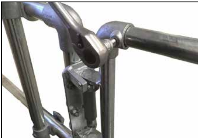
G. Disconnect the tubular gate from the hinge assembly by loosening the top & bottom cast clamp grub screw using a hex head socket as shown.
