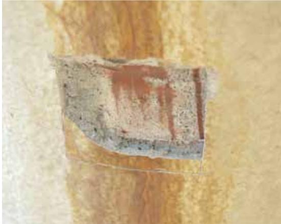
**Image: The *PITT-CHAR XP* coating intact with excellent adhesion and corrosion protection after 13 years in service offshore**
