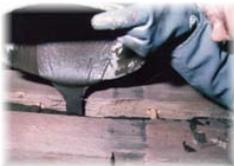
**COVERAGE:** When mixed both pack sizes of TG6 TIMBER GROUT will give the stated volumes of finished grout. As a guide, an 7.5 litre pack would fill a void of 100mm x 100mm x 750mm
