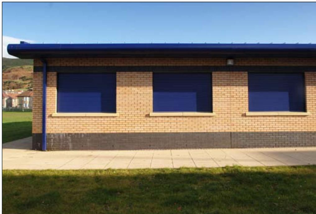
*The particular model of Charter-Integr8 shutter used at the Largs Academy allows the angle of the shutters to be tilted – just like a Venetian blind. This enables teachers to precisely control light levels in each classroom. The shutters were painted to exactly match the finish of the gutters, rain water pipes and windows – something which greatly enhances the building's overall appearance.*
