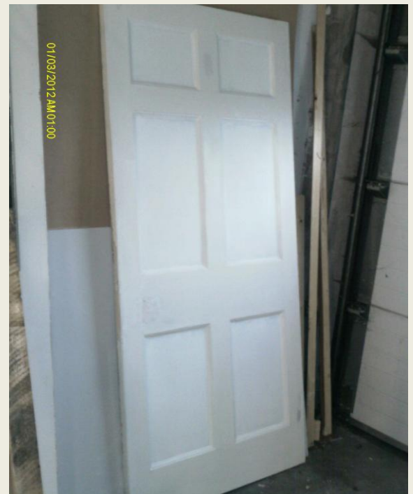
7: Stand aside and leave 24hrs to allow ITC coating to dry hard.
