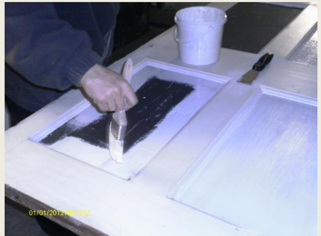
6: Apply 2 No coats Fireplug ITC to the whole leaf to ensure a uniform decorative finish.
