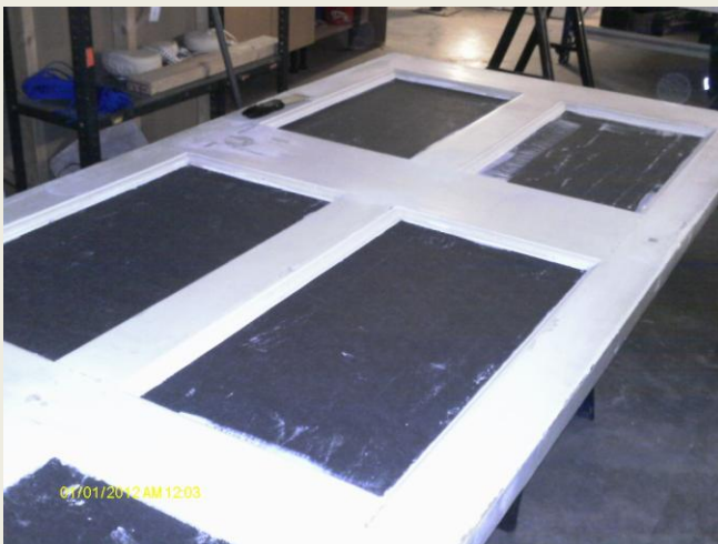
5a: Image shows all panels with membrane applied.
