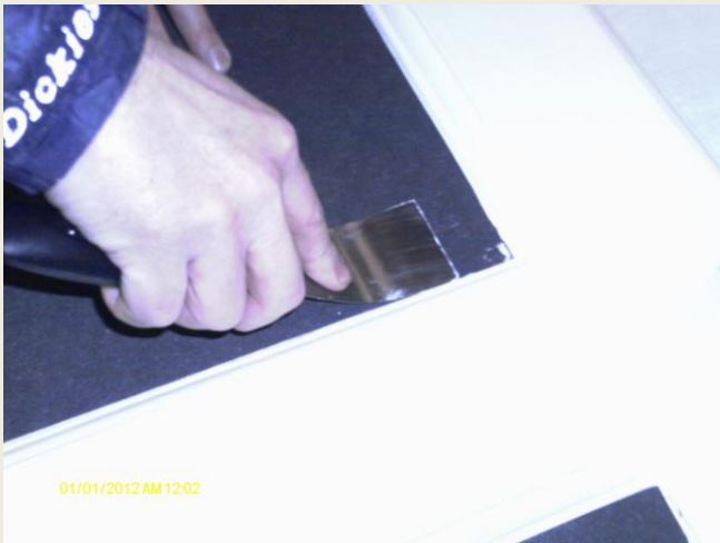
5: Using a flat scraper, flatten the membrane to the panel pressing in at all edges and at each corner. Take care not to leave air pockets.
