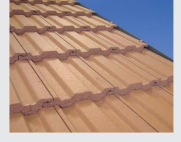
Fix using 2 x 25mm aluminium nails.
