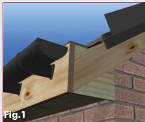
3. Slide the sprocketed connector onto the full length unit ensuring that the centre line of the sprocket connector is in line with the bottom of the eaves batten. Slide into the sprocket connector either a LH or RH short eaves sprocket length, (and seal with mastic), ensuring that the bottom overhangs the fascia by 50mm and nail to fascia.
