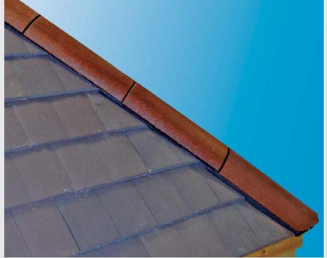
5. Position then nail a third round block-end ridge to the hip timber using 2 x 80mm screw nails and seals. Position and fix further carrier trays and third round hips in the same manner.
