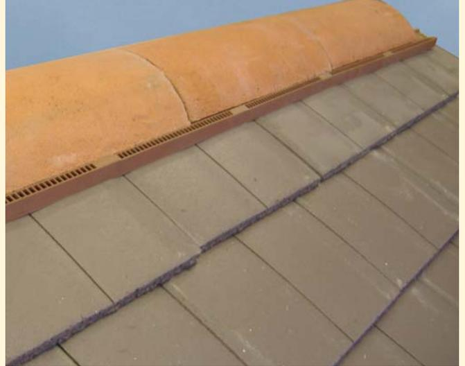
5. Place a block-end mono ridge at the gable end at the same time interlock two top fillers together locating them under the blockend. Secure the block end with 2 x 45mm 8 gauge s/s screws through the two holes in the vertical leg.
