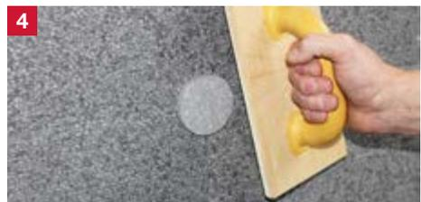
Using a float, or flat object to insert the *ejotherm* STR insulation cap flush with the surface - ready
