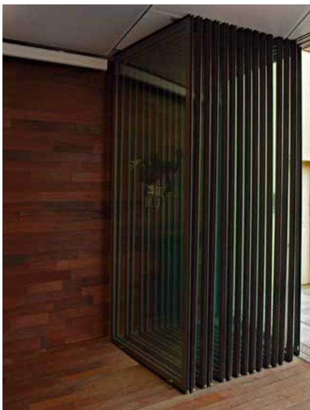
MSW stacking area, Pavillon Lapidarij Novigrad, Istra, Croatia (photo: Robert Les)
