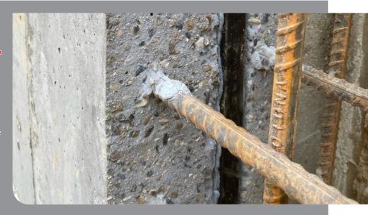
**Wykamol Gel Retarder** is a useful part of the **TT Admix System**, used to improve the concrete adhesion to surfaces by creating an excellent key. The gel consistency helps prevent run-off when applied to vertical surfaces and the blue pigment ensures adequate coverage across the substrate. This product can also be used with standard RC concrete.
