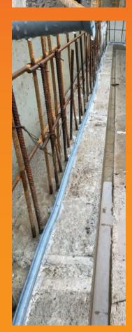
**WATERBARS** are a recognised joint sealing method in BS8102:2022, however waterbars must not be used in movement joint applications.
