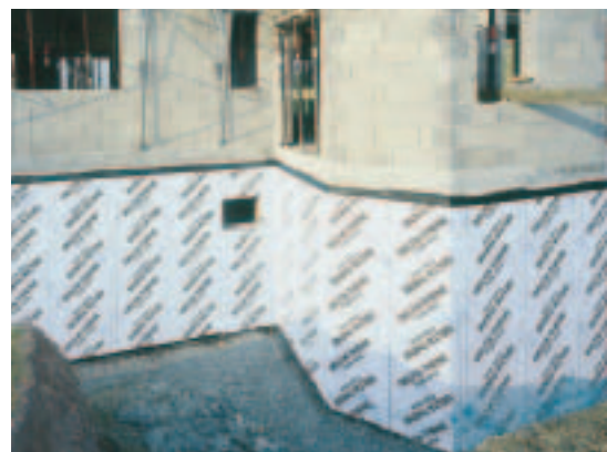
DELTA®-THENE is an excellent vapour barrier.
