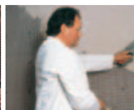
Simply apply plaster with a trowel.
