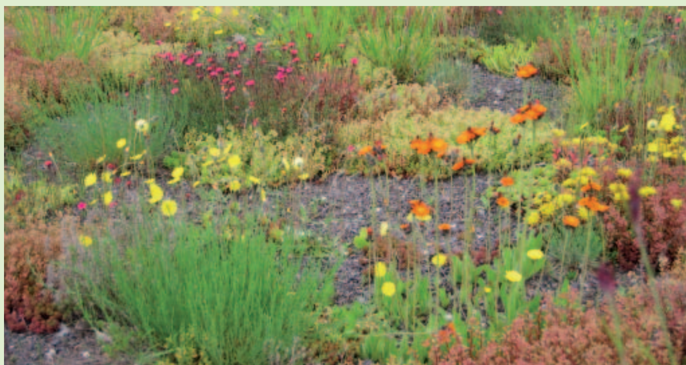
An extensive green roof
