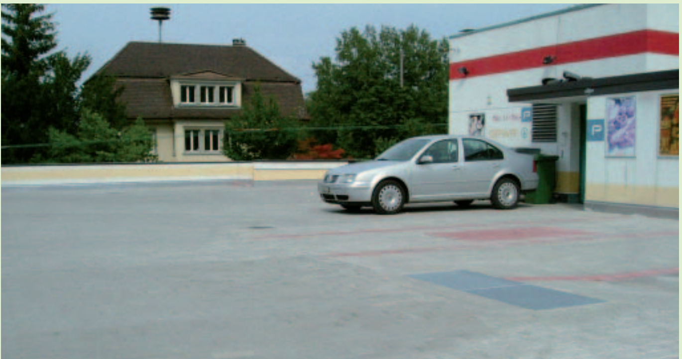
A drivable roof deck
