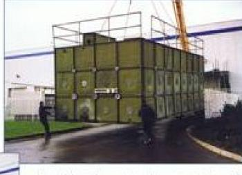
An old style sectional water tank with internal stay bars at a site in Shropshire.
