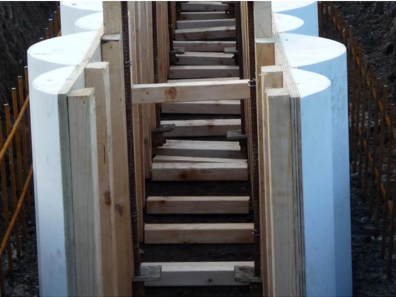
Cordek Reusable Guide Wall Formwork is used to accurately form an insitu concrete guide wall which is critical in the positioning and alignment of piles in a contiguous and secant piled walls.
