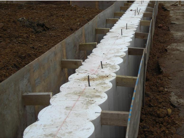
Sacrificial Guide Wall Formers are used to accurately form an insitu concrete guide wall which is critical in the positioning and alignment of piles in a contiguous or secant piled wall.
