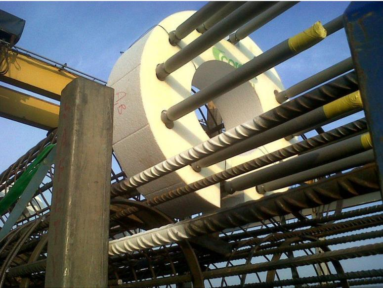
Corbreak is a unique system to aid the trimming down of piles. During the construction of piled foundations, it is quite often necessary to reduce the height of the piles and expose the reinforcement within them. The removal of concrete required to do this has been traditionally carried out using hand held tools which subject the users to a number of health and safety related issues e.g. noise and vibration.
