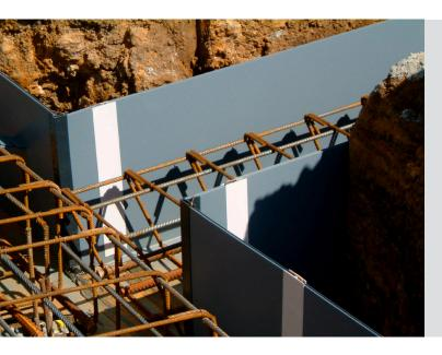
Sideform permanent formwork offers a quick and simple solution for minimising concrete wastage during the construction of cast in-situ ground beams and pile caps.
