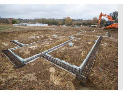
Heaveguard is a compressible expanded polystyrene product, used when foundations need to be protected against ground heave. As an integral part of the Cordek solution to ground heave, Heaveguard is used to protect against lateral heave, typically on the inside face of piled ground beams or deep trench fill foundations.
