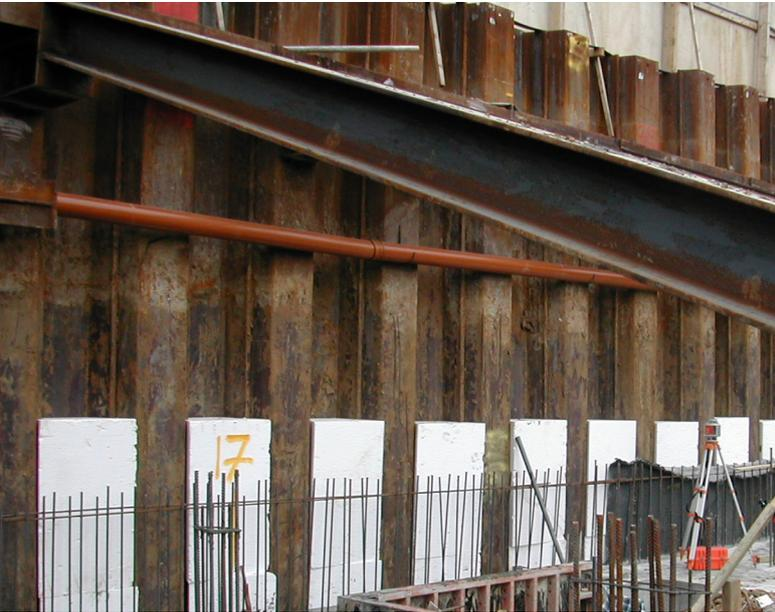
Sheet Pile Infills are designed as a quick, economical and lightweight solution to infilling the open pans in an exposed sheet pile wall. Manufactured to order from Filcor (Expanded Polystyrene), they are available in a range of profiles and densities to suit customer requirements.
