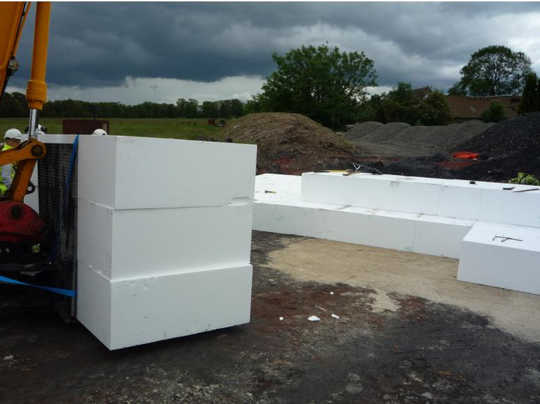
Filcor (Expanded Polystyrene) is increasingly being specified for an ever-growing range of applications. The most common applications include use as a lightweight structural fill alternative to more traditional fill materials or as a lightweight void former in structural concrete.
