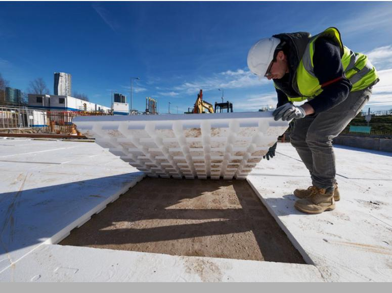
Ventform Plus provides an excellent passive gas venting medium under suitably reinforced concrete ground floor slabs with the additional benefit of incorporating below-slab insulation. When used in combination with perimeter vent outlets and a suitable gas resistant membrane system, it will provide an effective method of protecting structures against the ingress of harmful ground gases.
