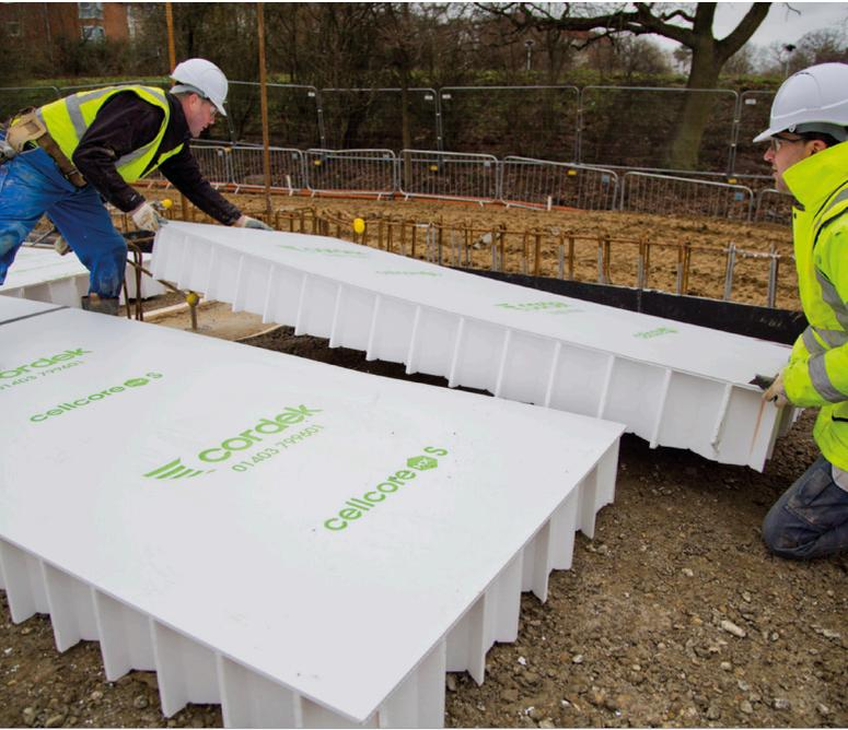
Cellcore HX is Cordek's fourth generation collapsible void former and has been designed to protect foundations from the effects of ground heave.
