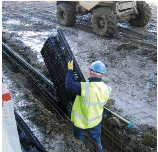
Lightweight unit, installed by one single worker.
