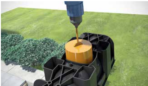
Produce connection openings.
