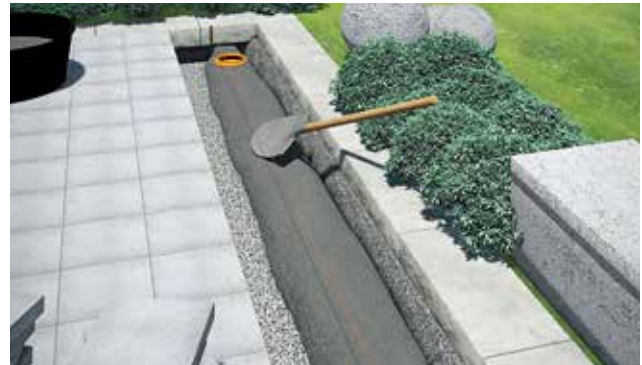
Fill with concrete and compress to foundation.
