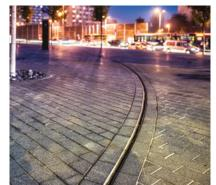
\*The A-symmetric slotted cover can be used along building facades, walls and landscape features at ground level.
