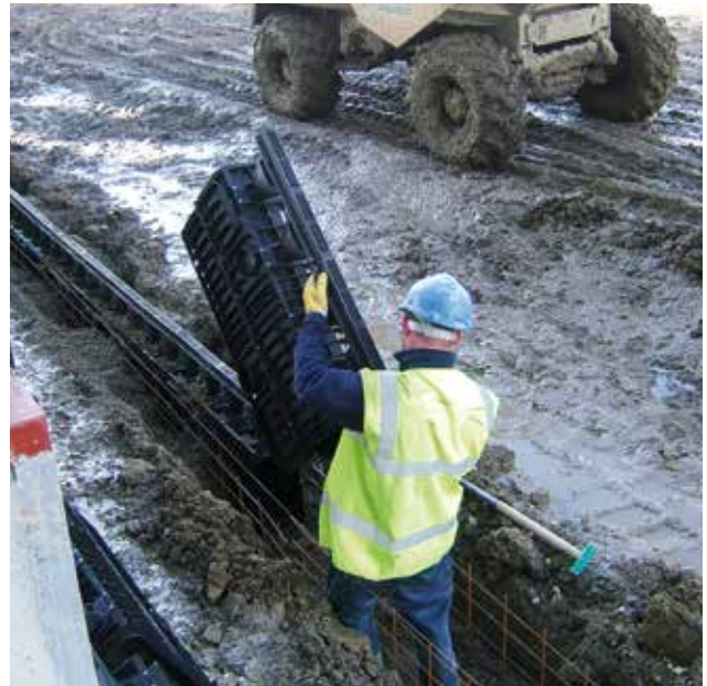
Lightweight unit, installed by one single worker.
