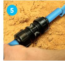
Push the fitting fully on to the pipe until the pipe goes right through the fitting.
