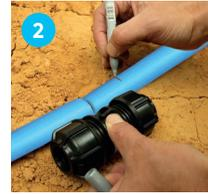
Lay fitting against pipe with damaged section in the middle of the fitting body. Witness mark against outer edge of nut.
