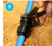
Tighten both nuts fully with a wrench or multi-grips until the nuts meet the flange of the body.
