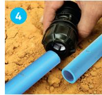
Push the fitting on to the pipe.
