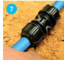
Move fitting until it meets the witness mark on both pipes.
