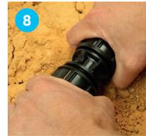
Tighten both nuts by hand.
