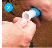
**Insert liner in PE pipe**
