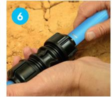
Bring the fitting back up to the pipe and over the damaged section.
