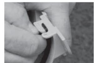
Using a notching tool, RGN1 (see page 31), notch the rear of the gutter. Notches must be made to both ends of a length of gutter.
