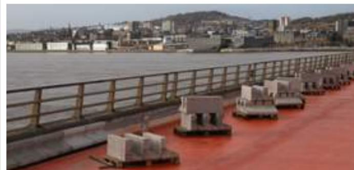
figure was 1.795 kN per metre of kerb therefore Brett Landscaping provided bespoke kerbs which were a maximum width of 336mm to enable the units to be below the required mass. This solution prevented the need to narrow lanes, thereby maintaining optimal traffic flow and safety on this heavily trafficked route in and out of Dundee.
