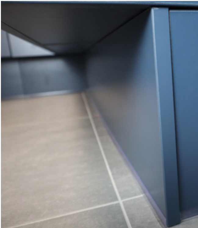
Recessed back and raised plinth height accommodates wheelchair footplates to increase turning space in kitchen
